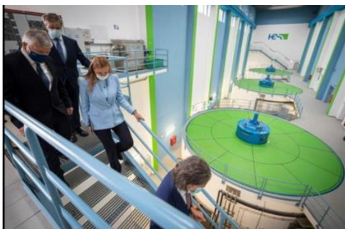
Kadri Simson (centre), European Commissioner for Energy, visiting a new hydroelectric plant in Brežice, Slovenia, 20 September 2021.
