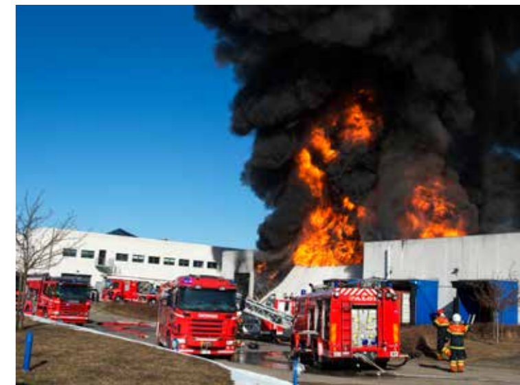
Tagbrand i industribygning under renovering med plastbaseret isolering. Roof fire in industrial building under renovation with plastic-based insulation. Foto, KJMFOTO/Kenneth Meyer
