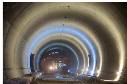
Tunnel T1 during construction
