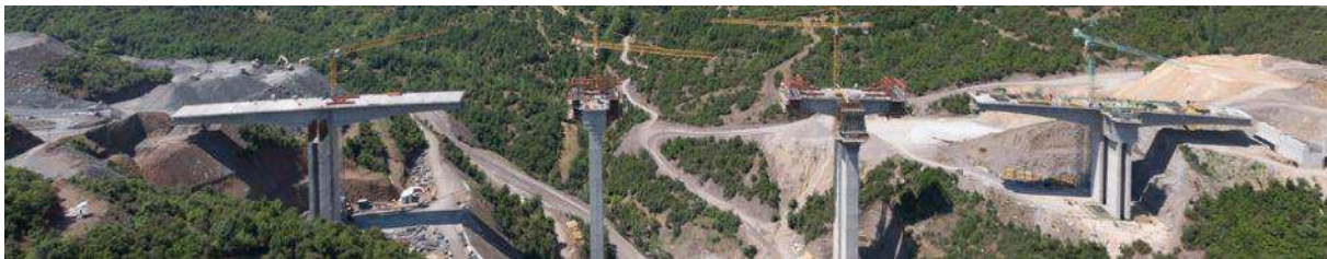
Bridge B3 during construction
