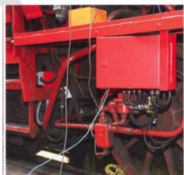
Figure 16 – Close up of the central unit 10
