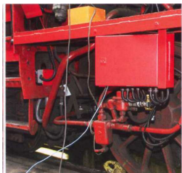
Figure 24 – Close up of the central unit 14
