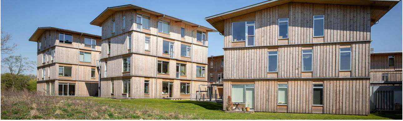
Project: FBAB Lisbjerg for Al2bolig. Architect: Vandkunsten. Photo: Helene Hoyer Mikkelsen
