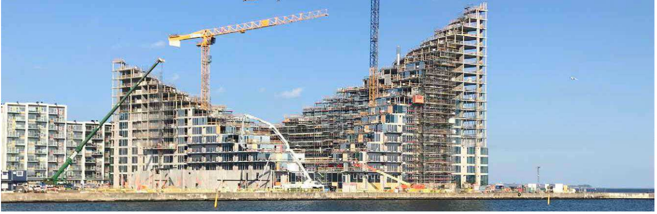
Multi-story housing construction in the Port of Aarhus.
