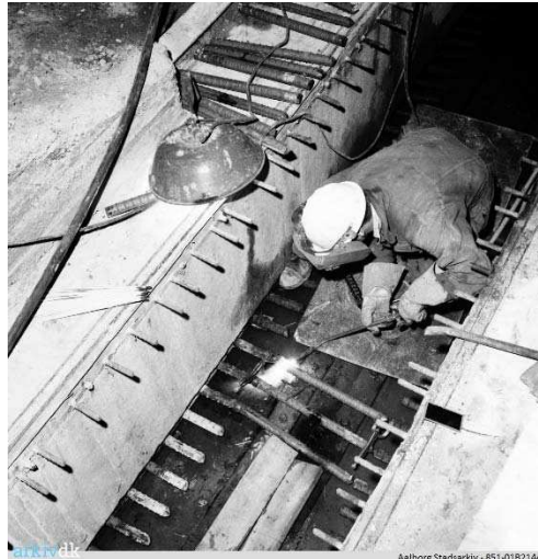
Figure 4.3-8 Immersion joint. The joint shown is between elements III and IV where additional reinforcement was installed due to the not perfect alignment.
