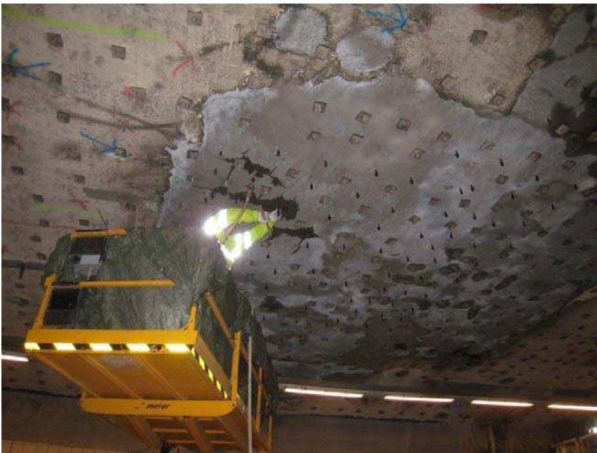
Figure 4.5-4 Injection of leaking cracks
