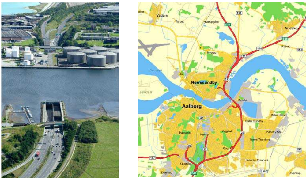
Figure 2.1-1 Aerial view and location plan considering the tunnel between Aalborg and Nørresundby.
