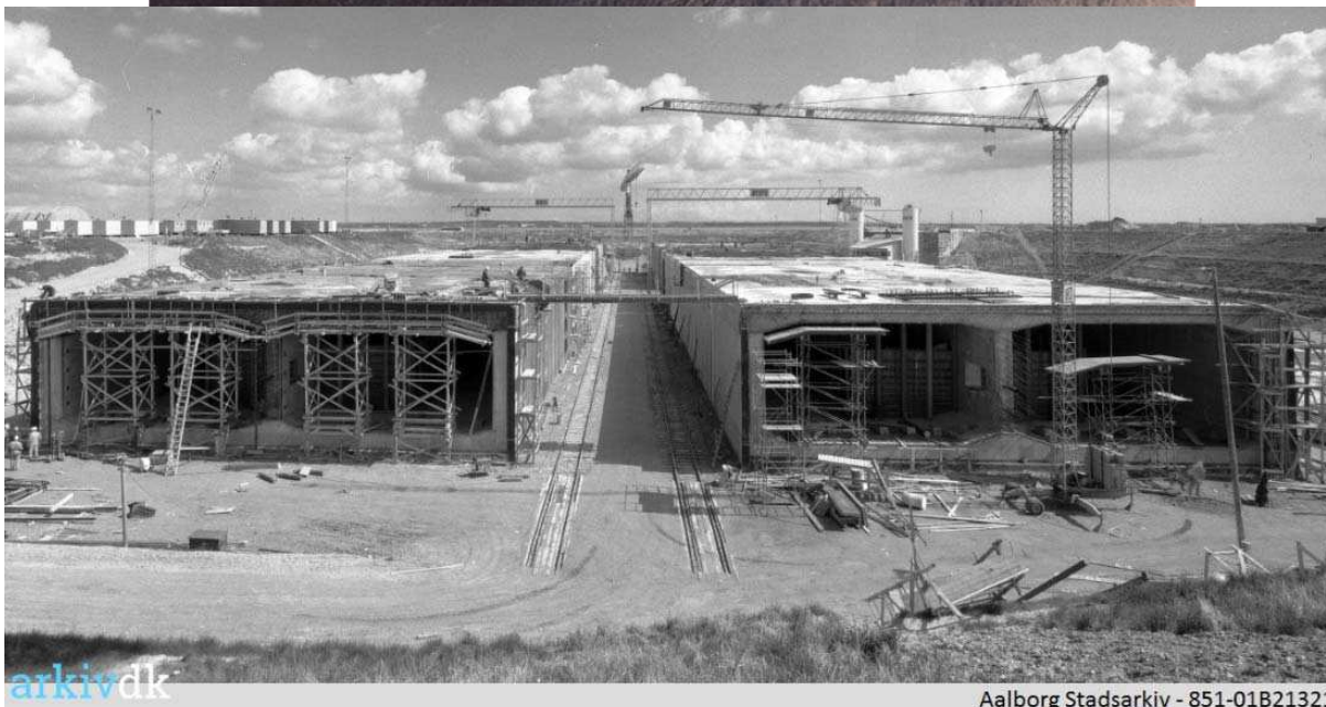
Figure 4.3-6 Casting of tunnel elements in the dry dock. The casting sections and openings can be seen on top picture.
