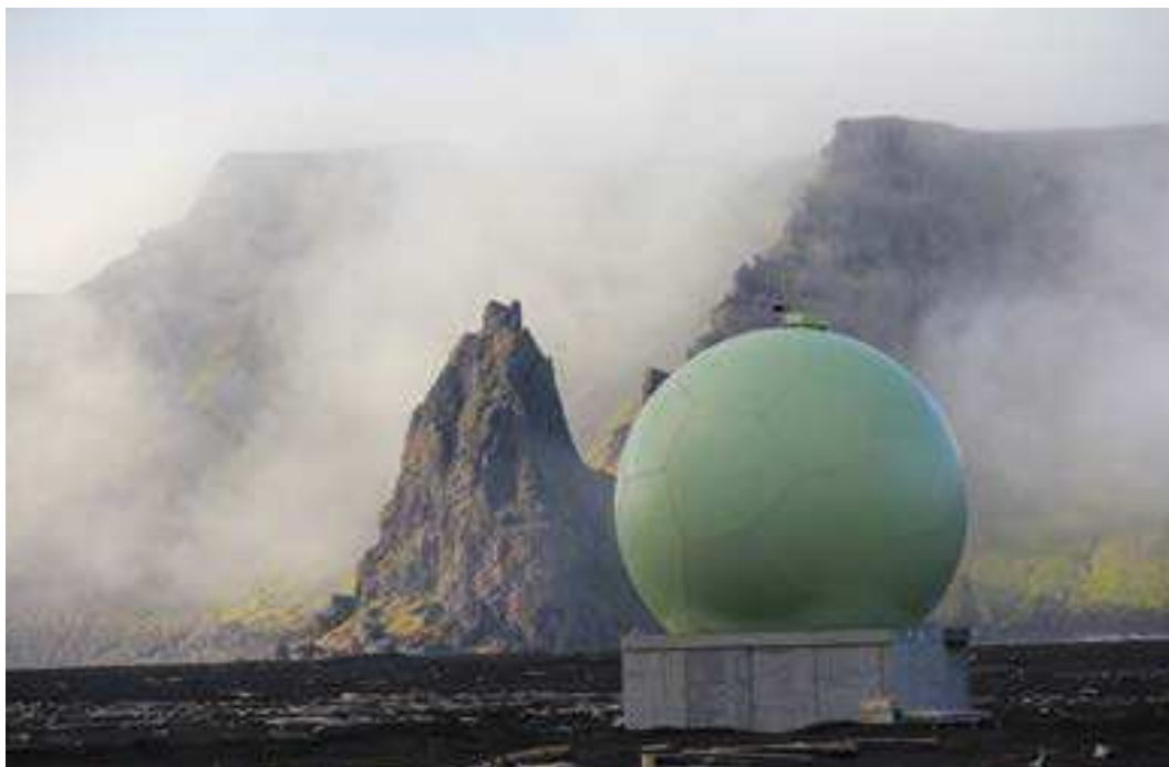
Galileo ground station on Jan Mayen Island in the Norwegian Arctic with protective 'radome' housing. The site houses a Galileo Sensor Station plus satellite link to pass data back to the Galileo ground system.
