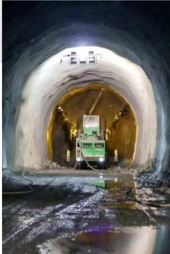
The explosives drilling truck
