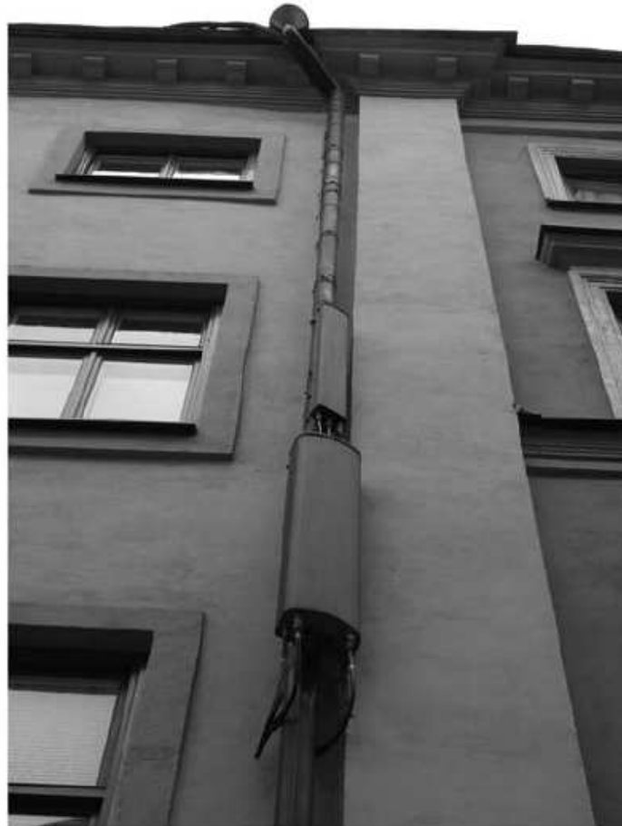
Figure 12. Stockholm Old Town measurement location with a relatively high radiofrequency radiation level, due to a mobile telephony base station antenna positioned at a low height and targeted towards the square.
