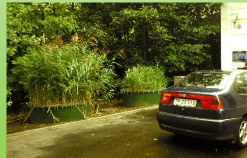
Carwash Water treatment
