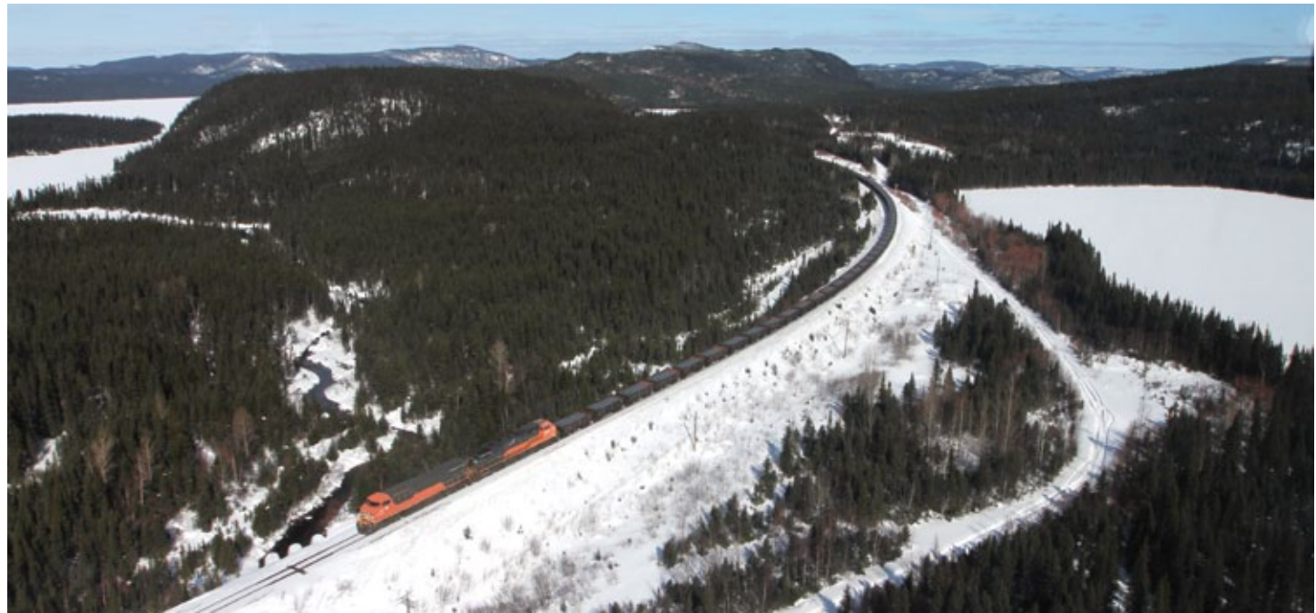
400km railway linking the mine at Mont-Wright to the harbour facilities in Port-Cartier. Photo credit: Arceor/Mittal Exploitation minière Canada s.e.nc.
