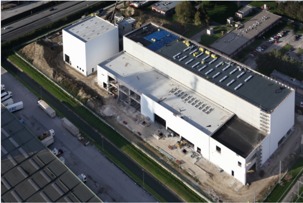
PRIMA building for the Neutral Beam Test Facility under construction at Padova in Italy
