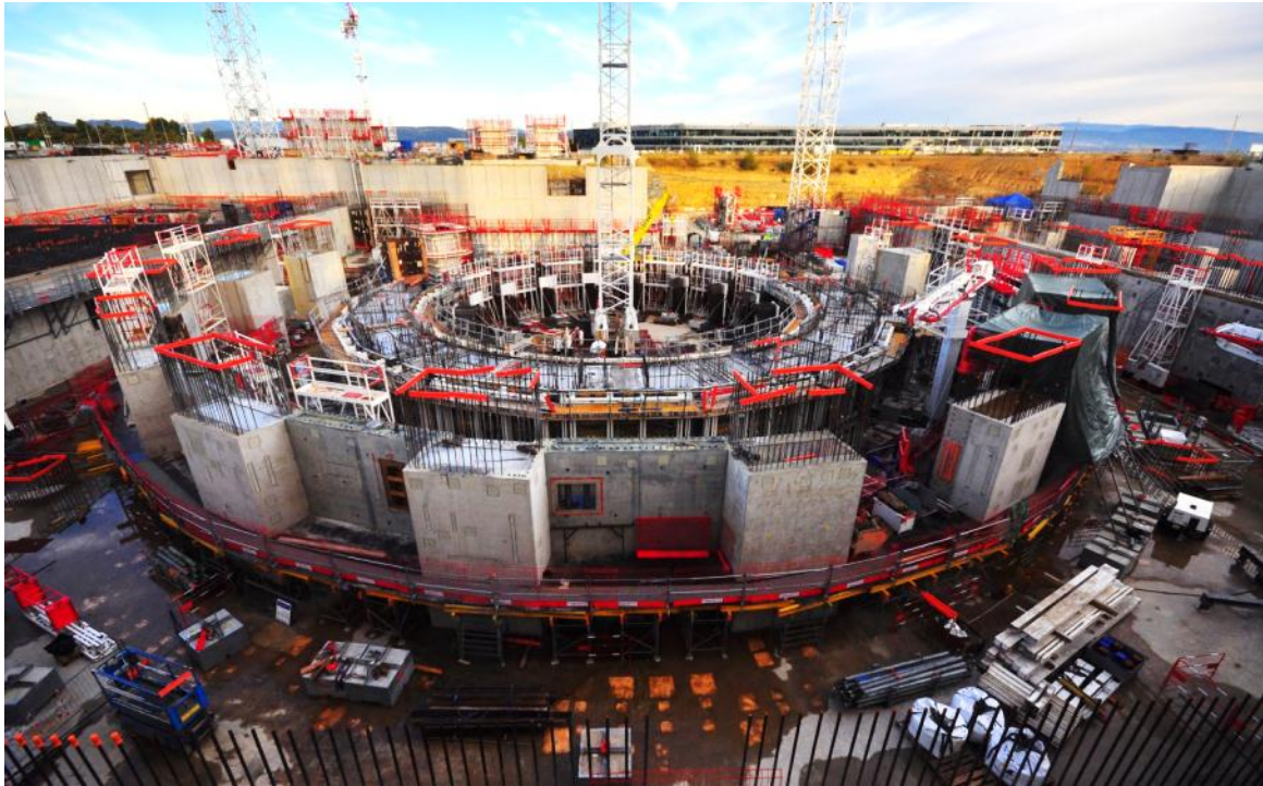
View of the central part of the Tokamak Building where the first half of the bioshield perimeter (a 200 degree segment) comprising some 620m 3 of concrete was poured in October 2015
