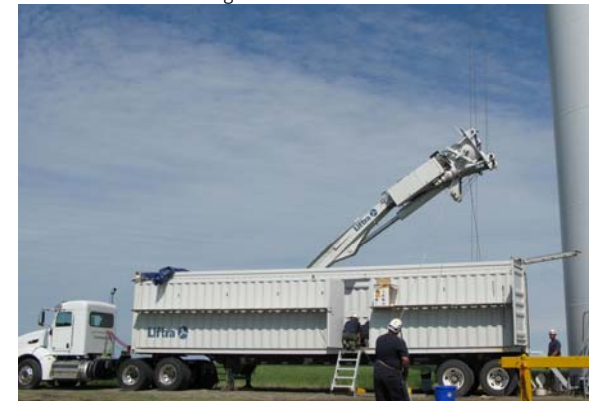
Liftra Self-Hoisting Crane climbing own lifting wire from container
