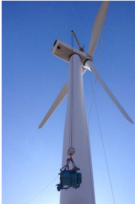
Lowering the gearbox to the ground
