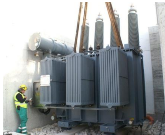
Installation of the insulating transformer for SPIDER and MITICA at the NBTF Site
