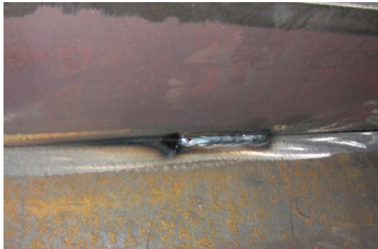
A tack weld from this project
