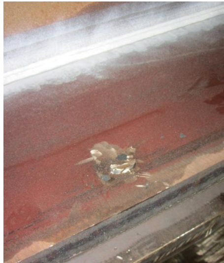
Surface irregularities are repaired
