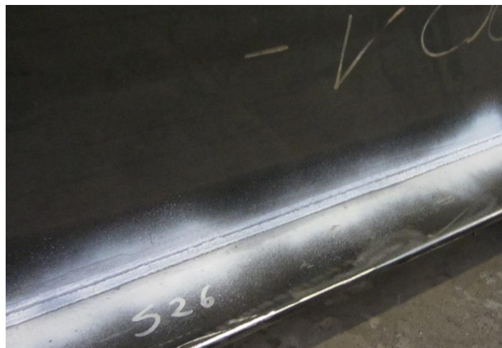
Traces after MPI testing.
