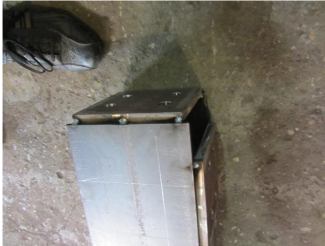
To short tack welds on profiles to another project
