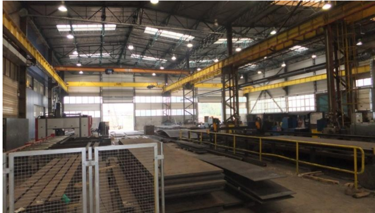
Shops with several travelling crane
