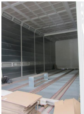
Separate paint shop
