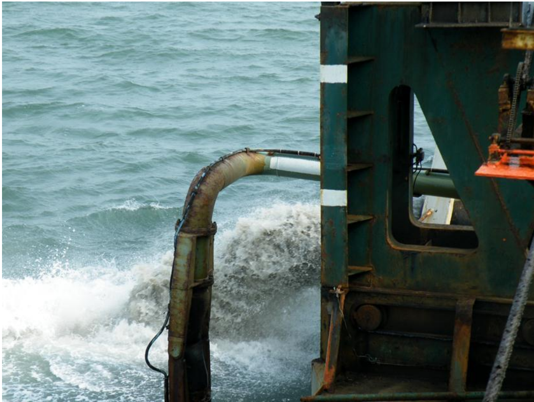
Water Injection to the dredging head
