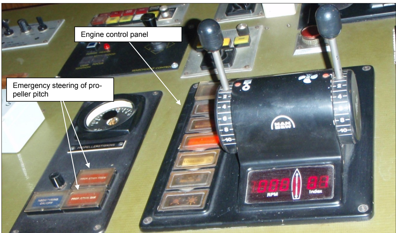
Figure 8: Engine control panel. Source: Private photo.
