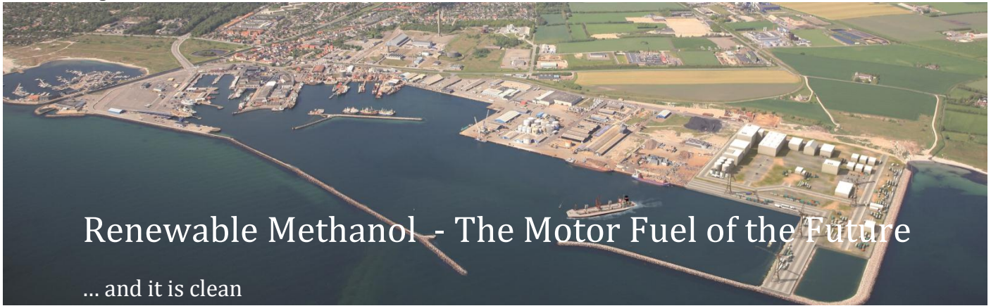
Grena Port. The upcoming fuel alcohol refineries (ethanol & methanol) will be located near the seaside.
