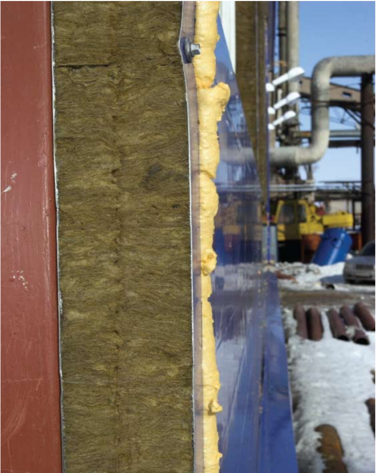
New insulation on boilerhouse in Russia
