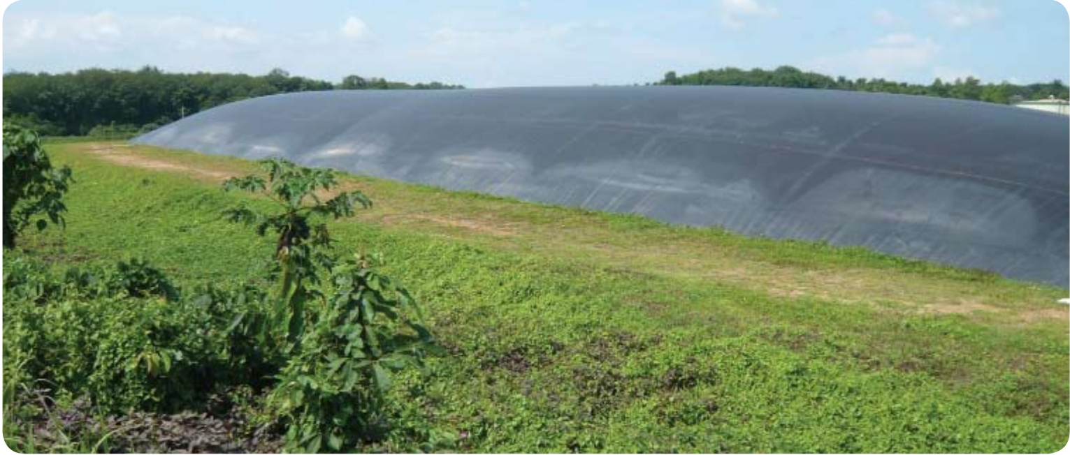
The membrane captures the methane gas produced from the wastewater used at the palm oil mill.
