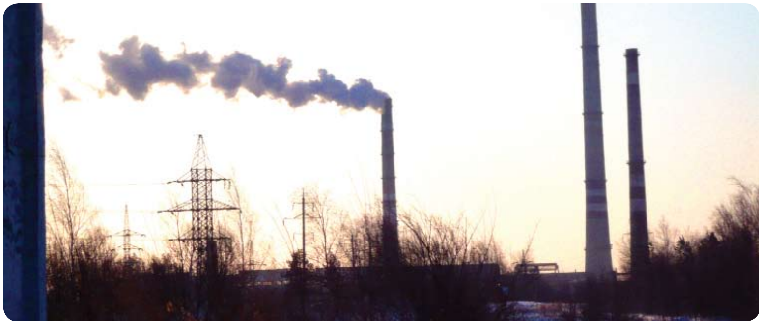
The essence of the project lies in modernization and switch from coal to natural gas in two of the boilers at the Amursk CHP.
