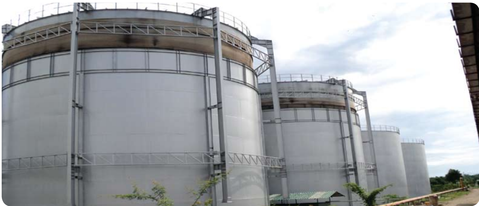
Biogas tanks at the Pinago plant. Methane recovery and utilization through the implementation of the project activity contributes to significant greenhouse gases emission reductions.
