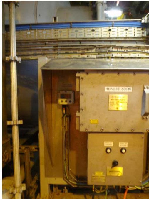
Figure A3.2 Continuous in-line Laser Induced UV Fluorescence Monitor
