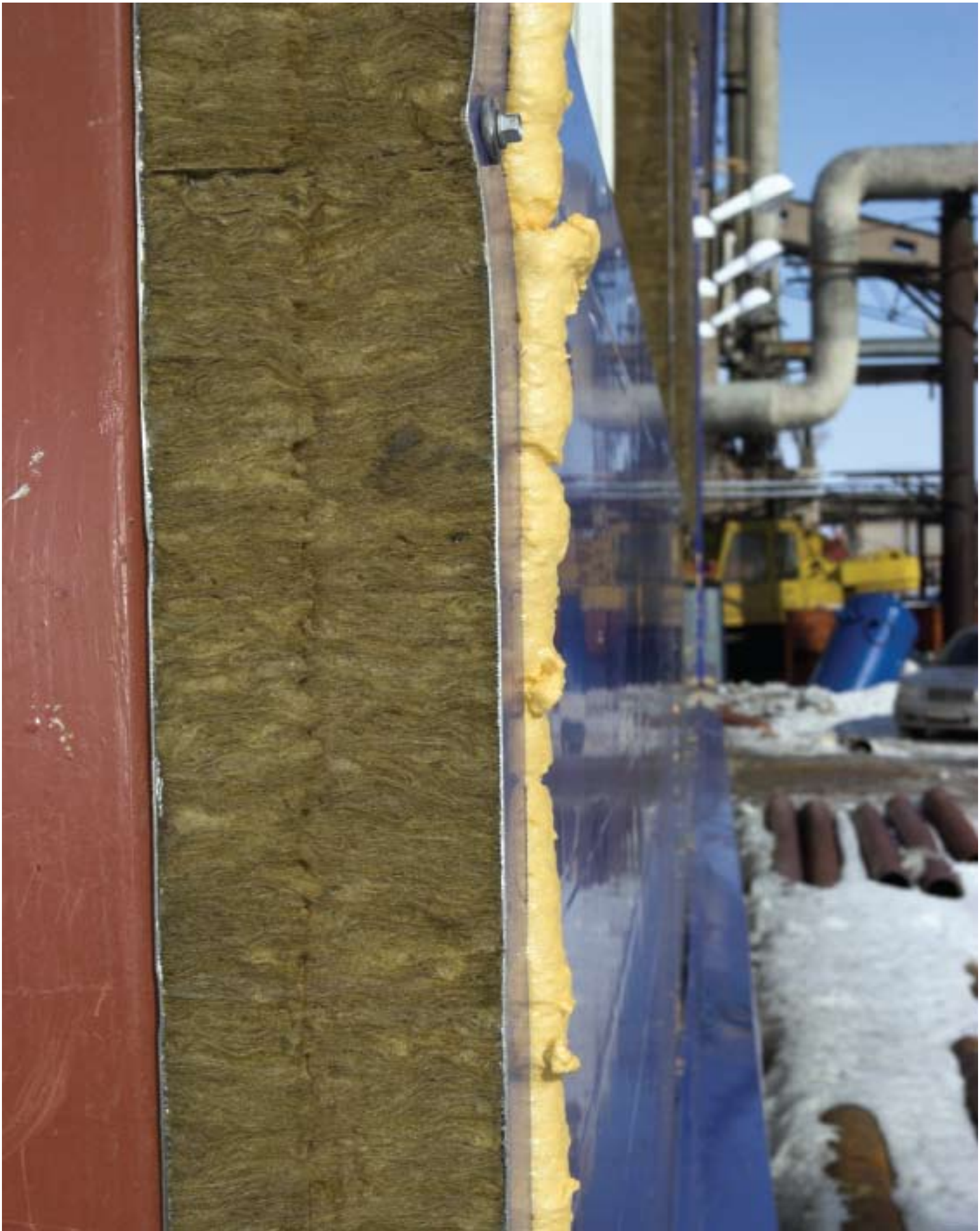
New insulation on boilerhouse in Russia
