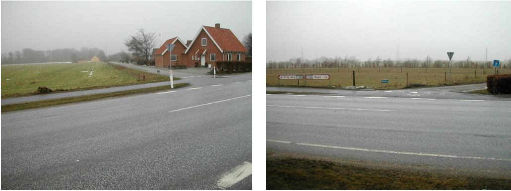
Figure 14 : Minor intersections on Road 150. Their unavoidable presence is the source of potential issues of charging equity.
