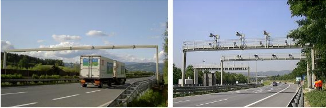
Figure 5: DSRC gantries and OBU in Austria (left: DSRC only, right: DSRC and enforcement).
