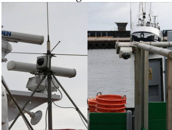
Figure 3. Photograph of an installed CCTV camera on a vessel encased in a cast aluminum armored dome.
