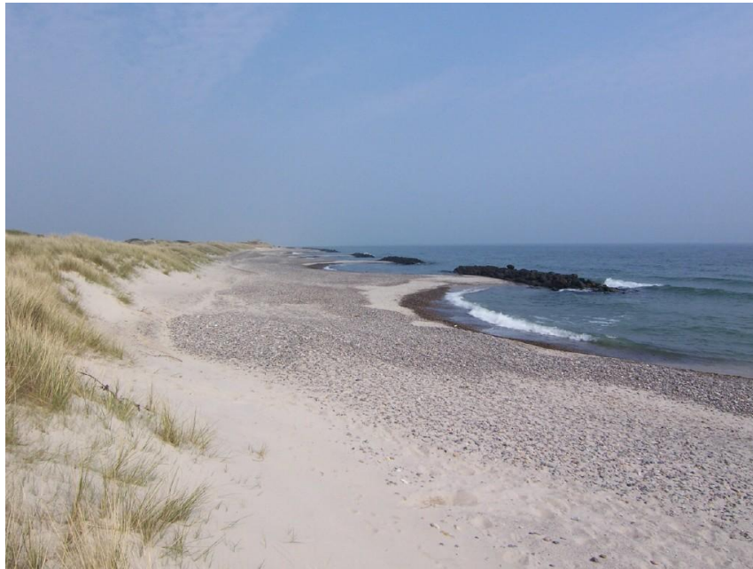
Fig. 58. Example of shore-parallel detached breakwaters. (Photo Hans F. Burcharth).
