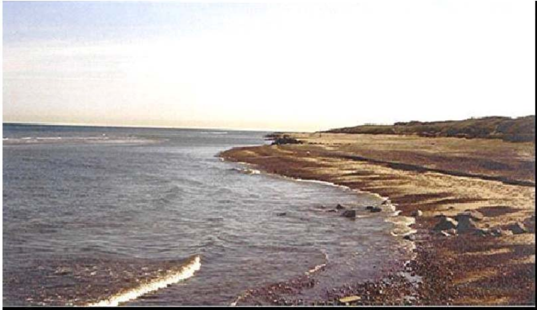
The PEM modules create a groin that catches long shore sand transport.
