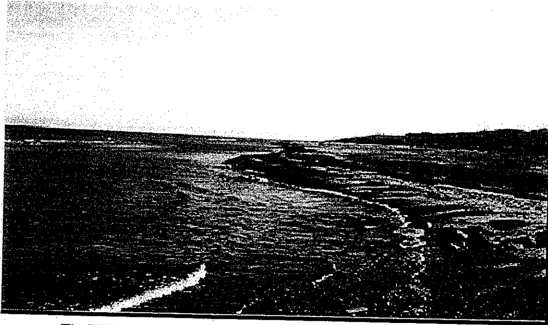
The PEM modules create a groin that catches long shore sand transport.
