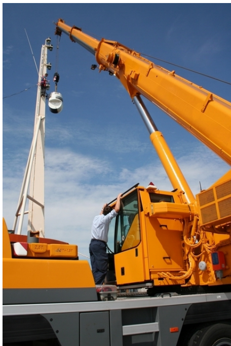
Sensor installation in the front mast
