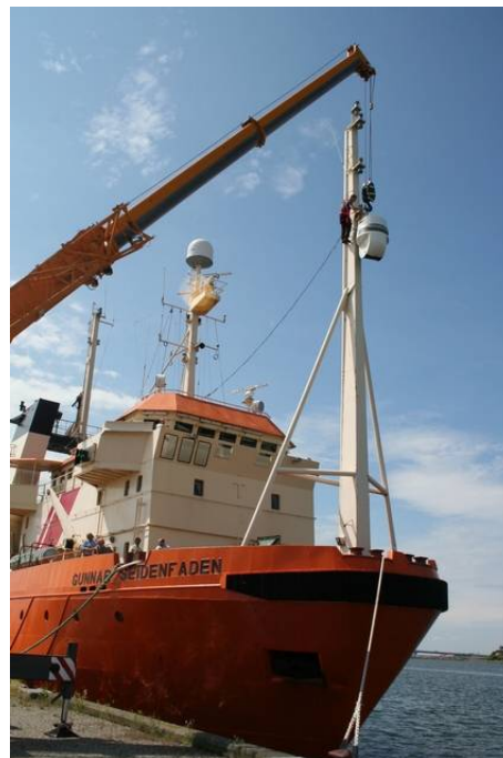
Sensor installation in the front mast
