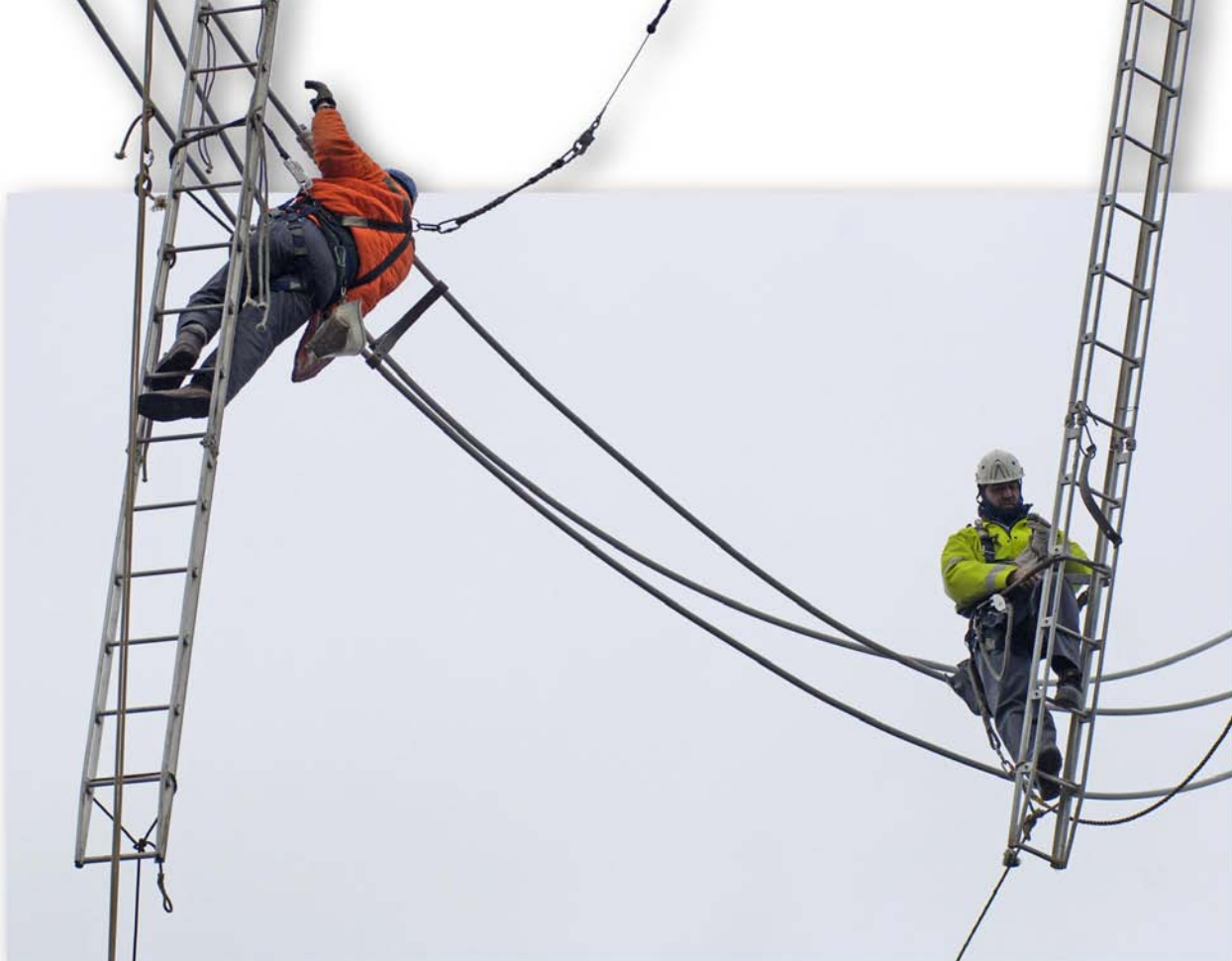
Work carried out on the 400 kV line Ulvila - Kangasala in South-Western Finland. Photo: Juhani Eskelinen
