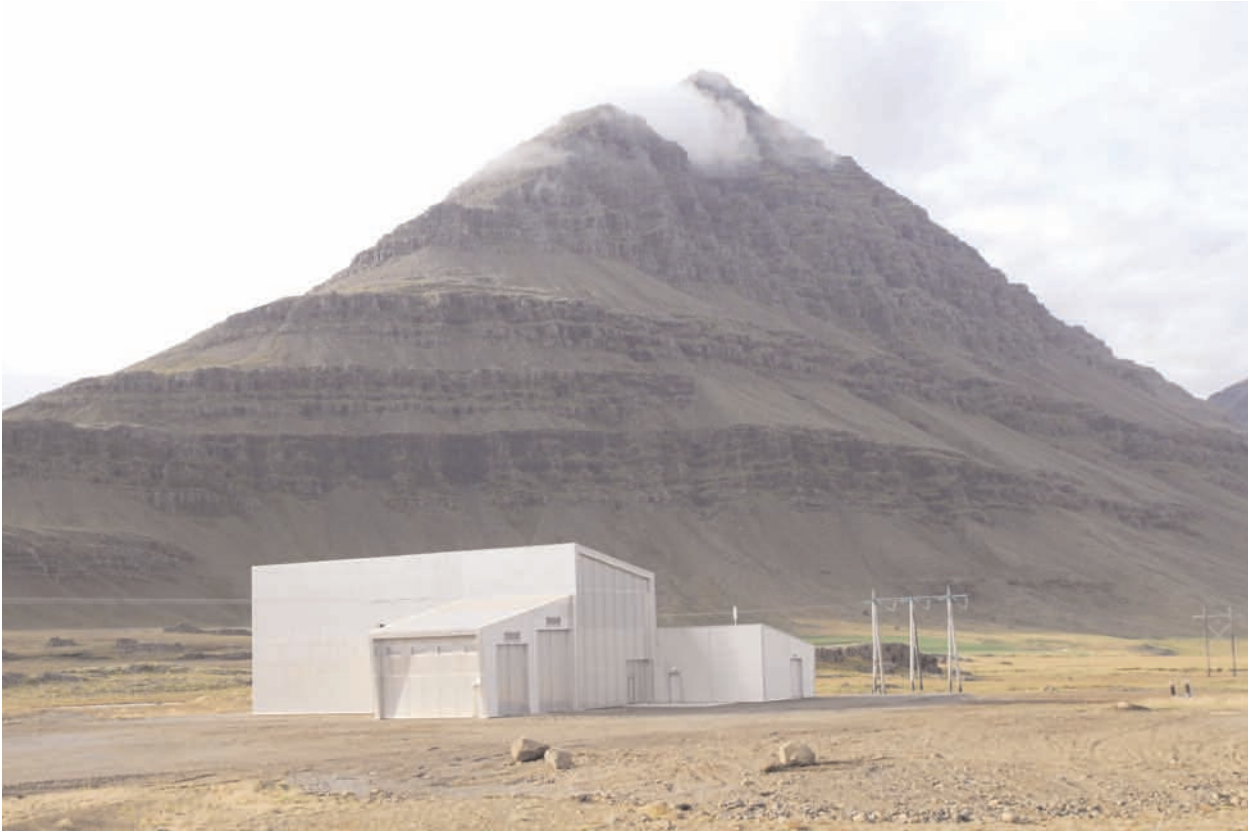
A new 132 kV substation at Teigarhorn in Eastern Iceland. Photo: Emil Thor
