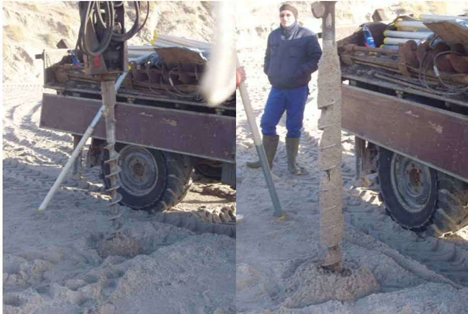
Figure 4.4A: Most of the tubes are installed by drilling, not to disturb the beach.
