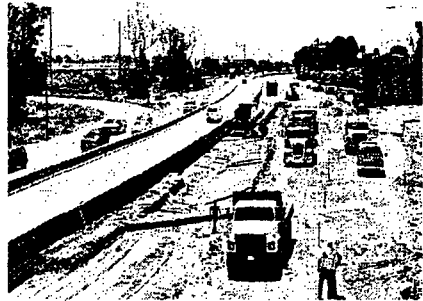
Digout and Placement of Aggregate Base – Working Platform
