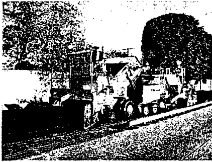
Placement of Leveling Course
