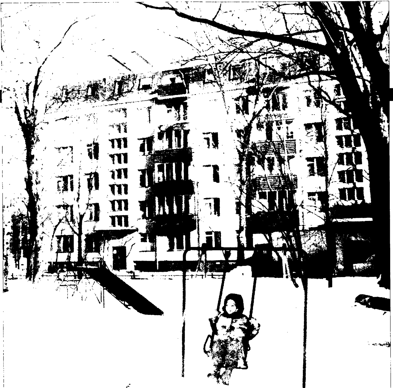
In 1999 Velux entered an apartment block renovation project in St. Petersburg, Russia, which involved installation of a new attic storey on the building
