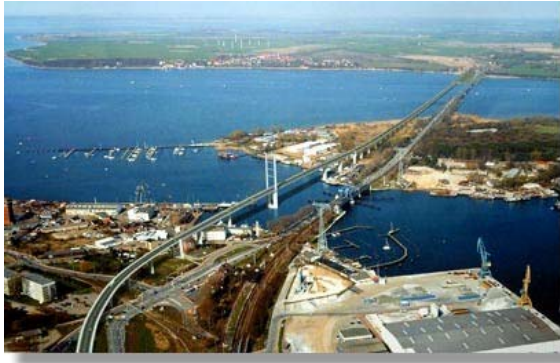
Picture 26: A computer animation of the new Strelasund Bridge with the present combined rail and road bridge on Rügendamm
