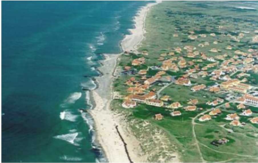
Fig. 11 Gl. Skagen PEM installation removed in 2001
