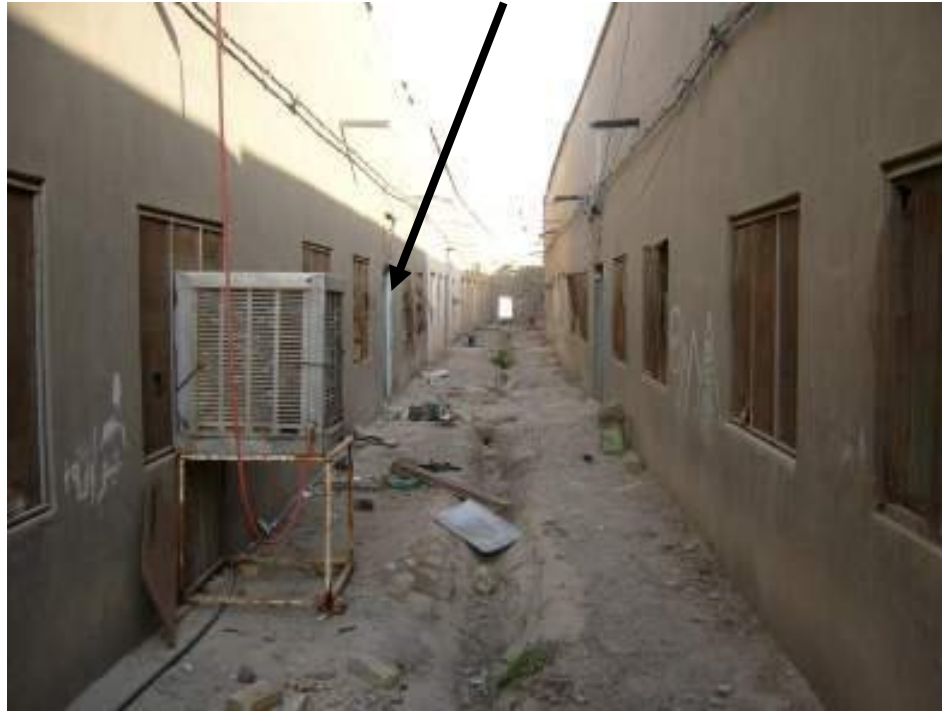
Facing North up the alley
